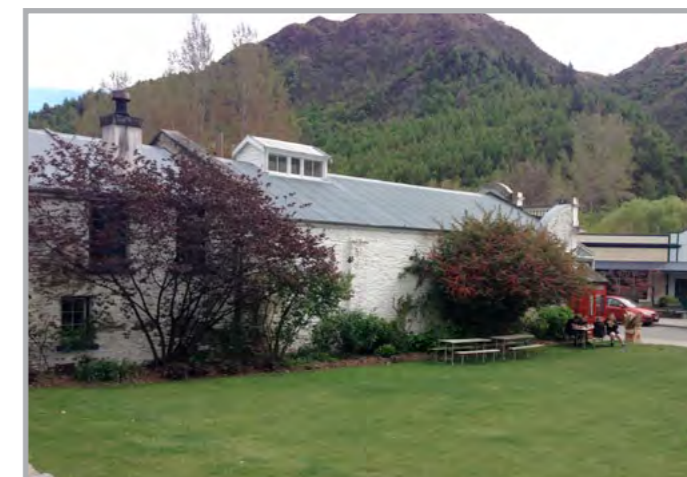
Uplights to stone wall on Pharmacy to create subtle backdrop for Buckingham Green
