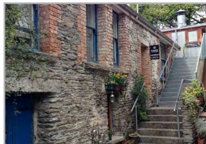
Assess current wall lights & highlight brick & stone features within Courtyard
