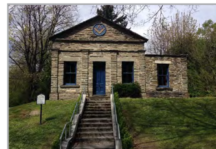
Uplights to facade, assess current lighting on entry steps
