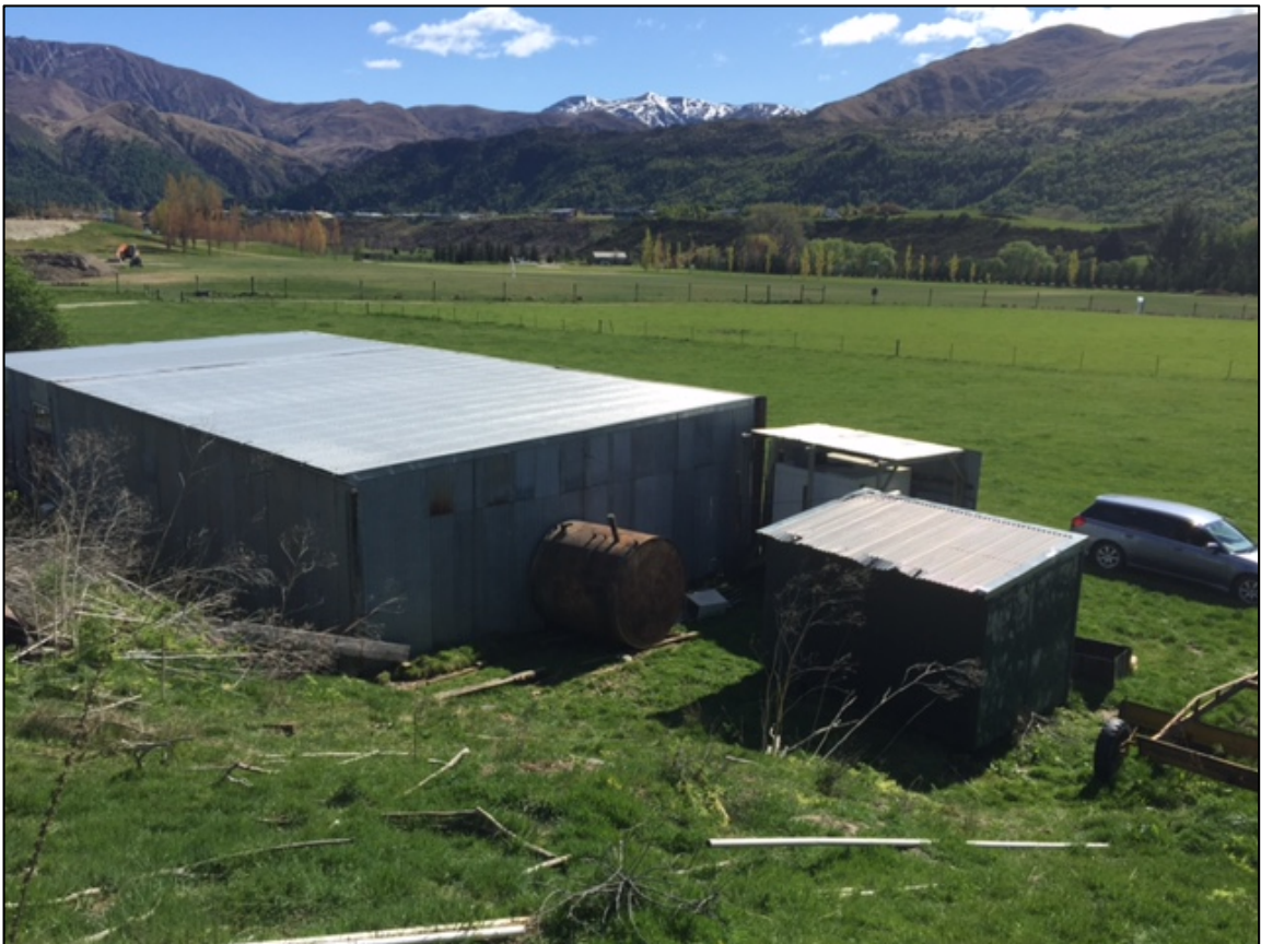
Plate 2: Behind hanger, looking north.
