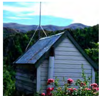
Small shed-out building.
