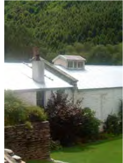
Side walls predominately solid.
