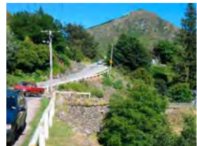
Butlers wall, Villiers Street behind.
