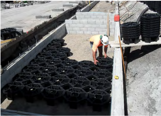
Integration of trees and infrastructure. Example of soil cells being laid out into tree pit areas. Image courtesy of Paul Malcolm, MetroGreen.
